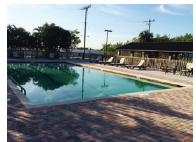
The restored pool at Air Station Miami.
